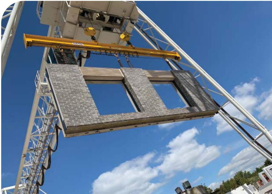
LEFT: A storey-high, two-room wide insulated precast concrete sandwich panel with reconstructed stone headers and cast on brickwork being made ready for delivery following installation of glazing at the factory.
