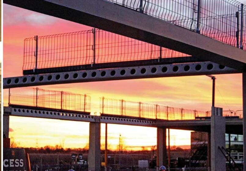
Composite Deltabeam steel section spanning between precast columns with safety barrier preinstalled.
