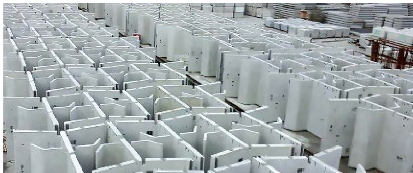
Offsite manufactured repeatable components in storage yard
