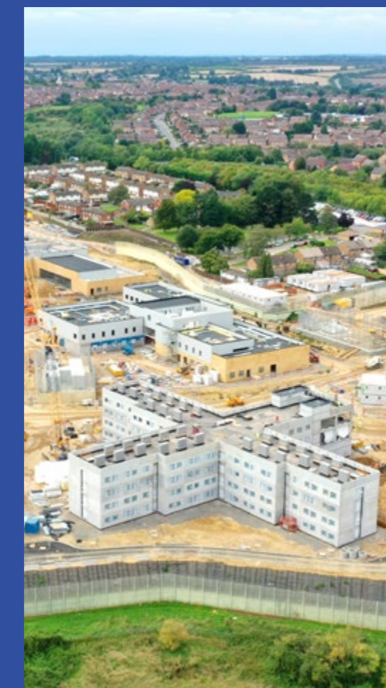
HMP Fosse Way in construction
