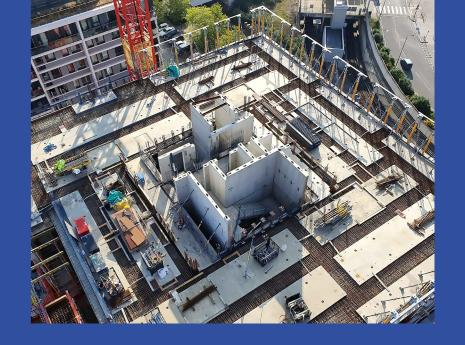
small changes to be made which aggregate to have a significant impact on the overall process. Simple changes such as preloading the flooring components with loose reinforcement positioned exactly where steel fixers need it, prefabricated shutters, reinforcement cages and pre-fixing edge protection prior to being lifted into place all contribute to improving site efficiency.
