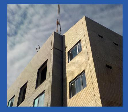
and Safety with reduced waste. Some of the facade panels also included structural steel sections cast in to facilitate the appearance of continuous glazing at the wrapround corners of the building.
