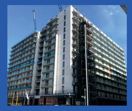
which 'see saws' over the structural external wall. This innovative idea allowed cantilever balconies to have the glass balustrades to be fitted offsite at a preassembly facility prior to the balcony being delivered to site and then assembled form within the building footprint resulting in the removal of external access and the risk of operatives having to access the outside edge of the structure.
