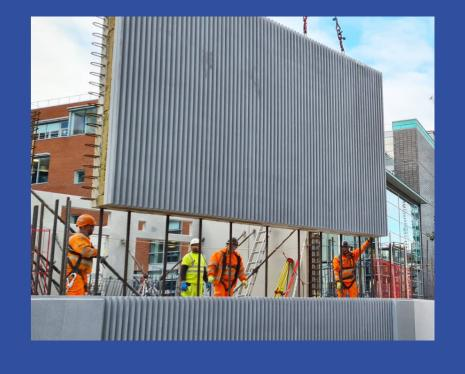
In all, some 44 architectural and sandwich panels, 200 tonnes of steel columns, 440 twin and solid walls, over 1,000 hollowcore floor units, 249 steel Deltabeams with 9,000m² of reinforced structural topping came together to showcase a first class PCE HybriDfMA framed office building for the centre of Bristol. Great importance had been placed by PCE's Engineers
